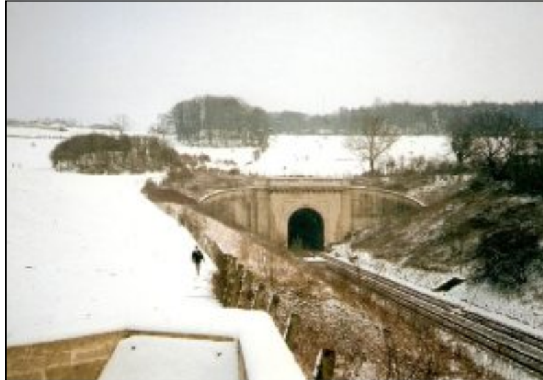
GOING UNDERGROUND: The Western Portal of the Box Hill Tunnel
